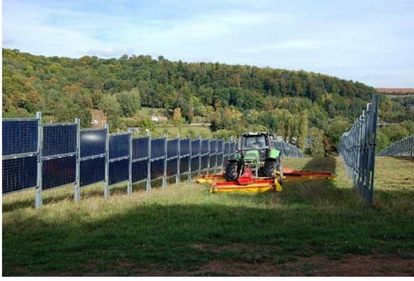
Fig. 1. Example of vertically mounted PV modules for AgriPV applications [9] (left), and for noise protection walls on highways [10] (right).
